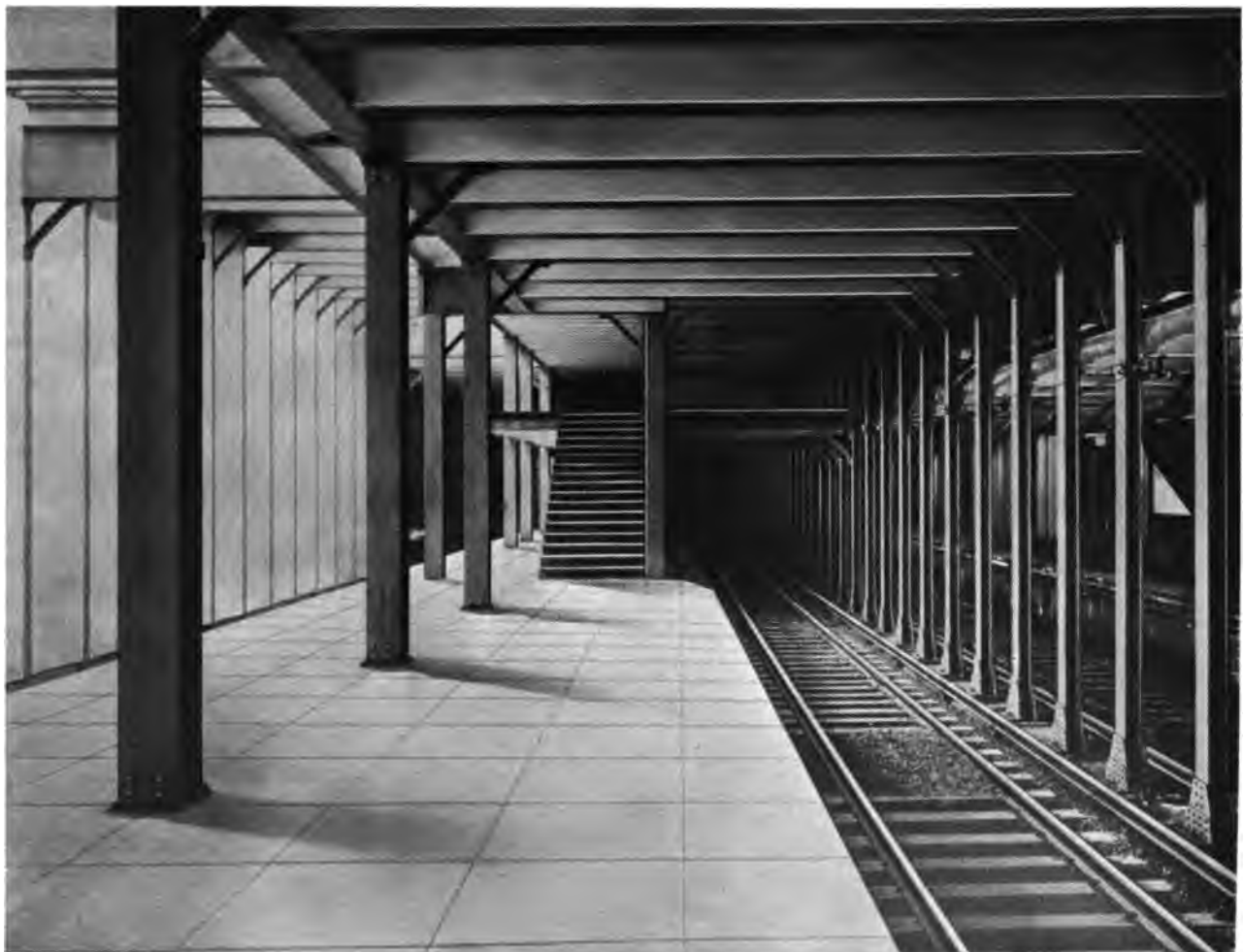
EXPRESS STATION AT 14TH STREET, SHOWING ISLAND AND MEZZANINE PLATFORMS AND STAIRS CONNECTING THEM
